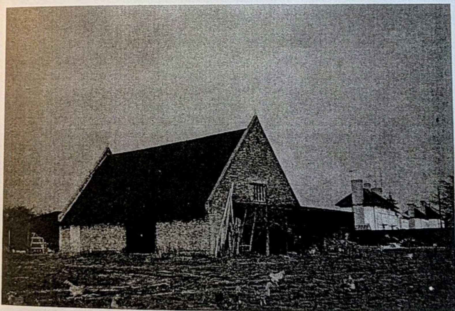
Red brick barn at Linden Farm; thatched roof was replaced with corrugated iron. Now a large domestic dwelling as part of the Rickyard Development in 2003. Note "free-range" hens in the fore ground.....No factory farming in those days!
