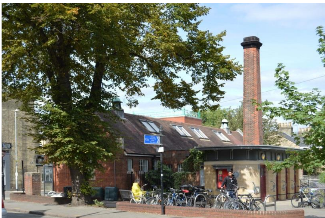
Figure 28 – View from across Mill Road looking at the southeast corner and the public toilets
