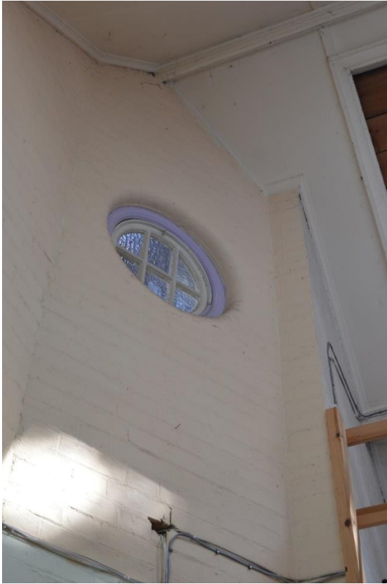
Figure 59 – Internal circular window
