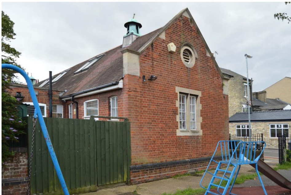
Figure 29 – View from the play area looking at the northern side of the building
