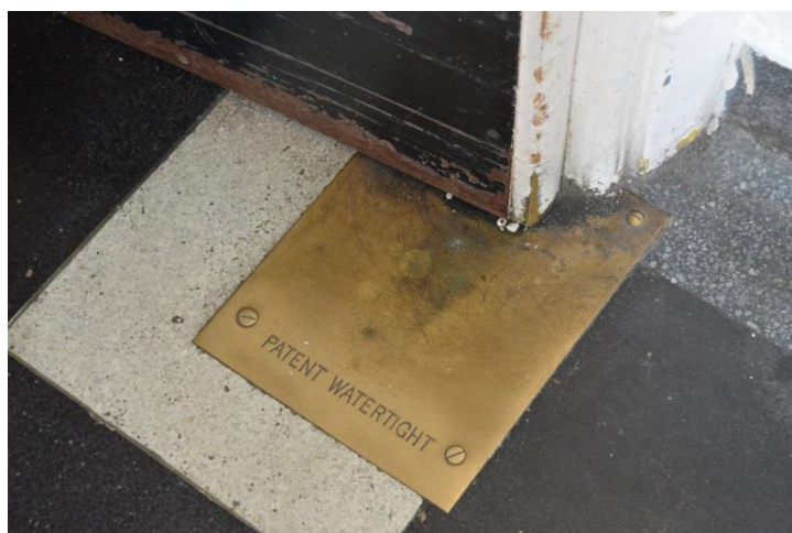
Figure 40 – Brass floor-plate from swing doors
