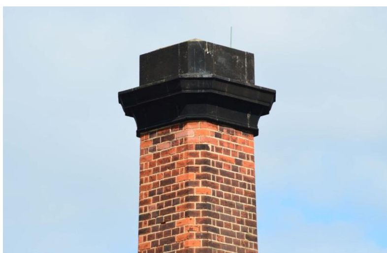
Figure 32 – Bath House chimney
