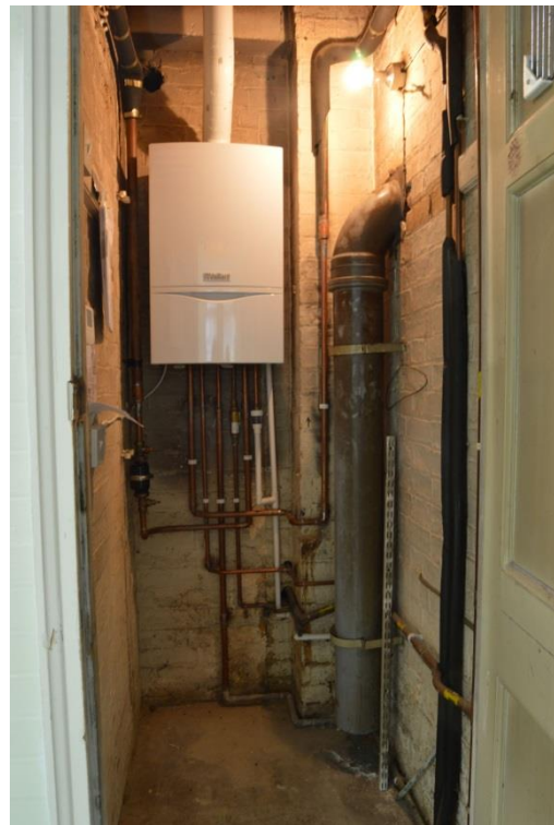
Figure 56 – Remnants of old boiler
