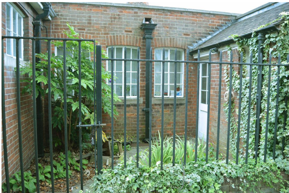
Figure 47 – Former laundry and drying room, exterior view
