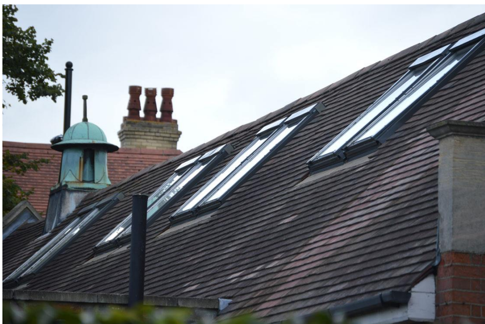
Figure 51 – Roof lights, exterior view
