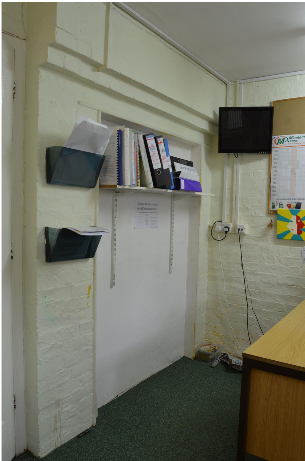
Figure 49 – Former access way to drying racks
